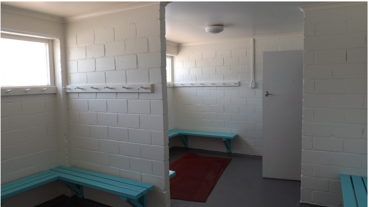
Figure 3: Internal view of building interior with internal masonry walls
